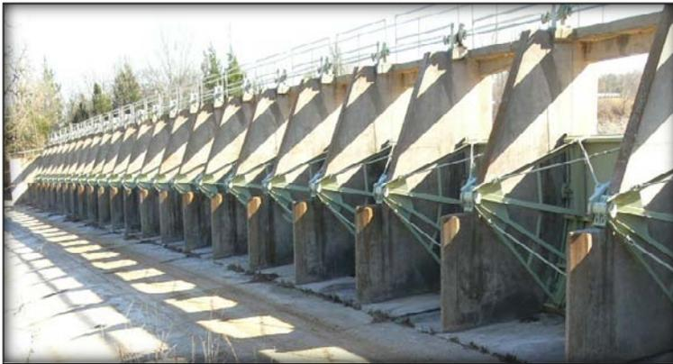
The dam has a spillway that consists of 23 small, manually operated radial gates and two fixed concrete ogee weirs. The gates are under design to be replaced by reinforced concrete ogee weirs with variable fixed crest elevations that will allow the dam to pass the TCEQ design flood. The fixed weirs will eliminate the need to use City staff to operate the gates during inclement weather.
